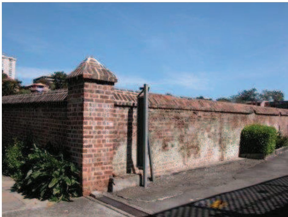
Figure 14 - St Johns cemetery boundary walling that extends around the site and creates the frontage to O'Connell Street (Source State Heritage Register entry)
